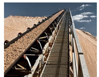
FAG split spherical roller bearing installed in a conveyor system
