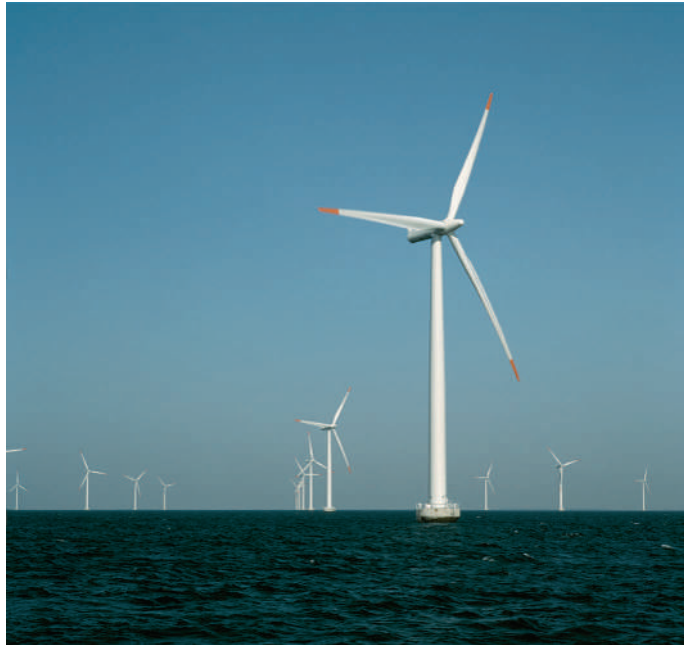
16 Application example, offshore wind turbine
