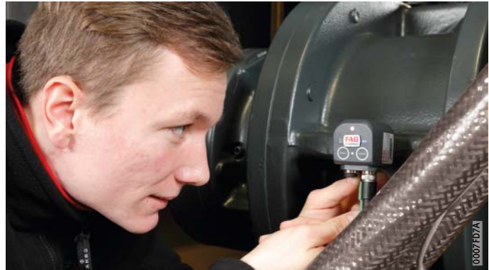
Figure 3 Commissioning of FAG SmartCheck
