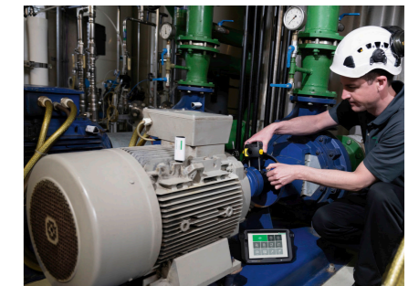
Industry: LASER-EQUILIGN2 always ensures professional alignment of your machines thanks to single laser technology
