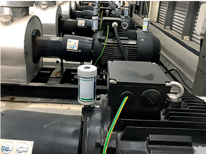
Industry: CONCEPT1 lubricates umpteen motors
