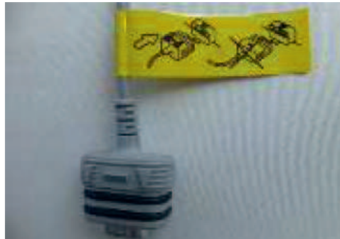
④12 Information signs for electrical operating switches
